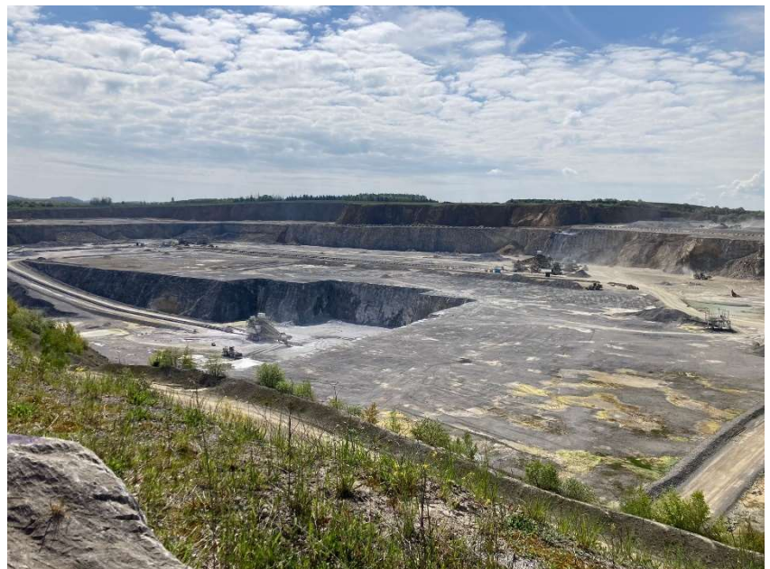
A section of the limestone quarry
